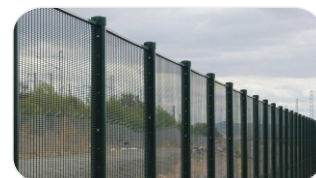
LAYOUT FENCING & DEMARCATION
