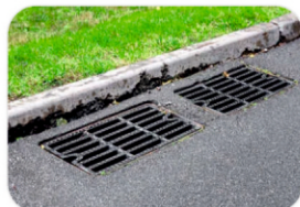
STORM WATER DRAINAGE
