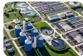
SEWAGE TREATMENT PLANT
